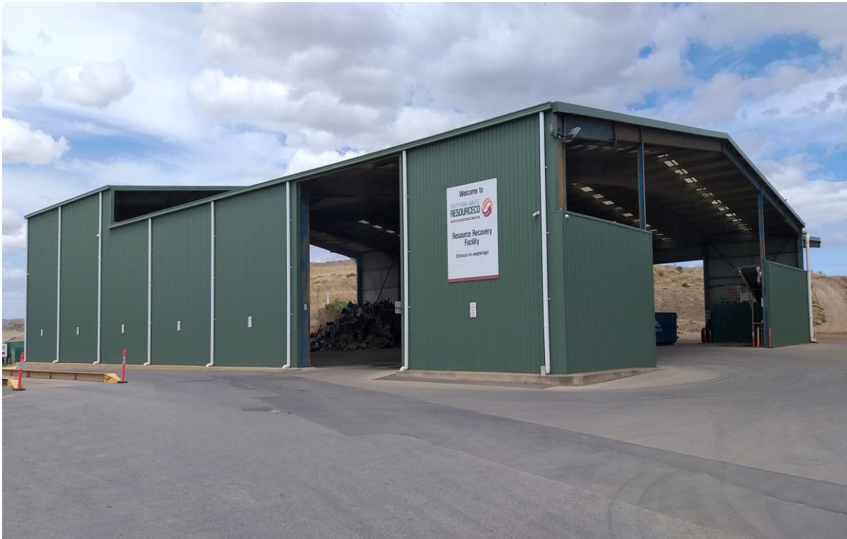
Figure 3 – Material Resource Recovery Facility
